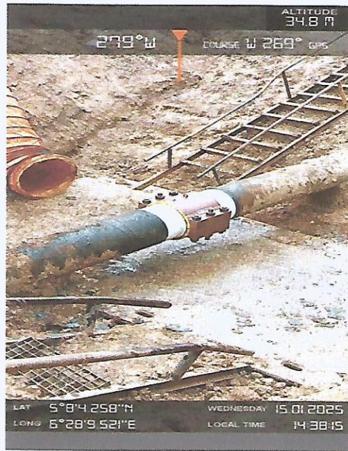
Fig 2. Showing point after repair.
